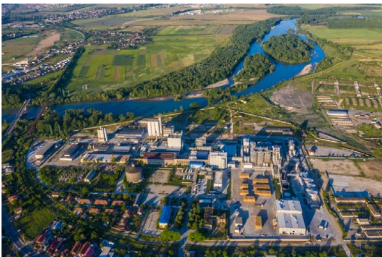
Clariant's flagship sunliquid® cellulosic ethanol plant in Podari, Romania. (Photo: Clariant)
