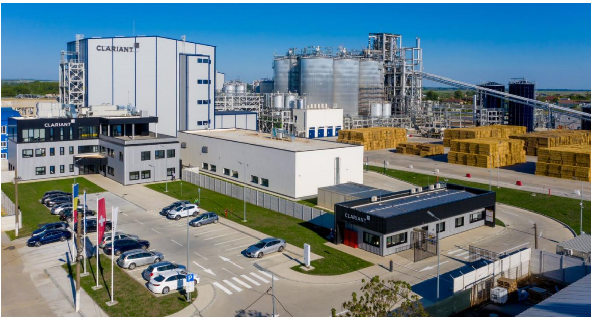
Clariant's flagship sunliquid® cellulosic ethanol plant in Podari, Romania. (Photo: Clariant)
